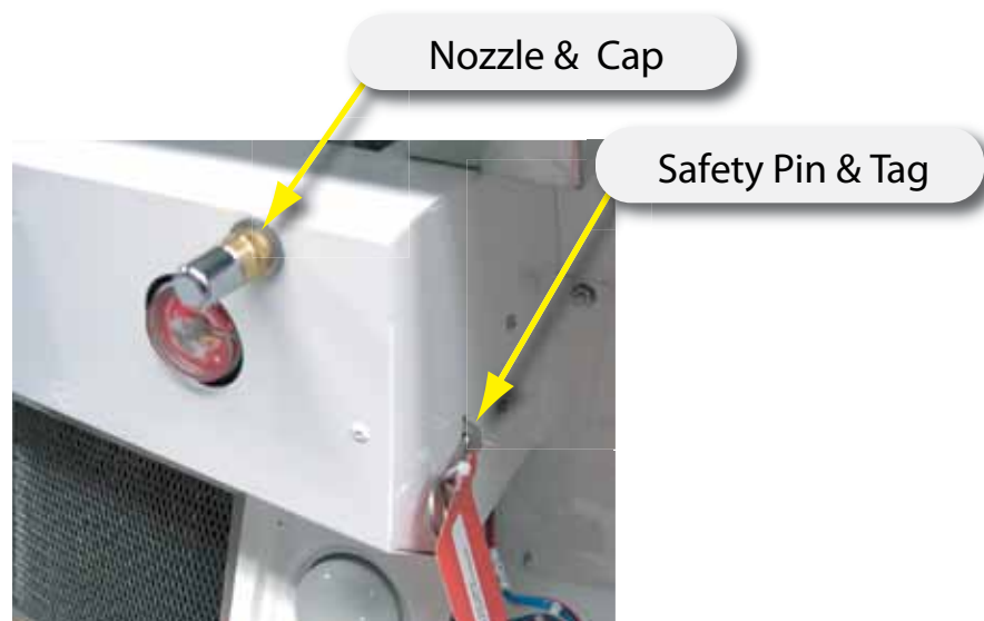
Tank Assembly - Safety Key and Nozzle Assy
